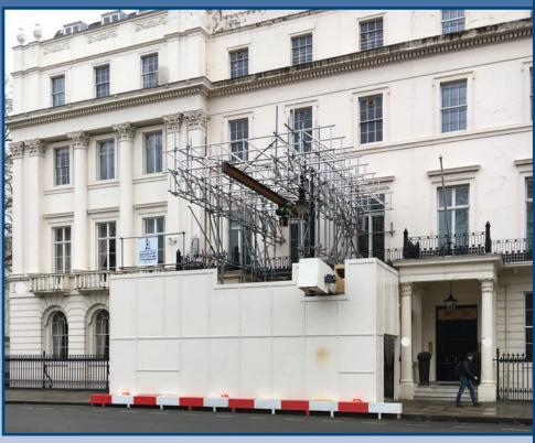
The project comprised of the construction of two levels of basement below the lower ground floor of the existing building. The basement level will include a fitness suite and the sub-basement level will accommodate an indoor swimming pool and associated plant rooms.
